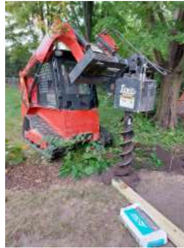
Drilling post new post holes →
