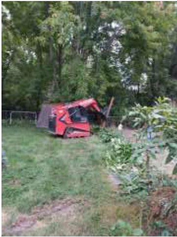
← Taking down the old fence
