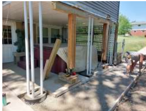
Forms are put in place & new concrete slab is poured.
