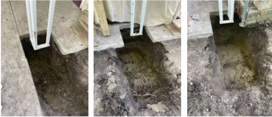
Above: Day 1/Some demolition to remove the old footing and the start of the new one.
